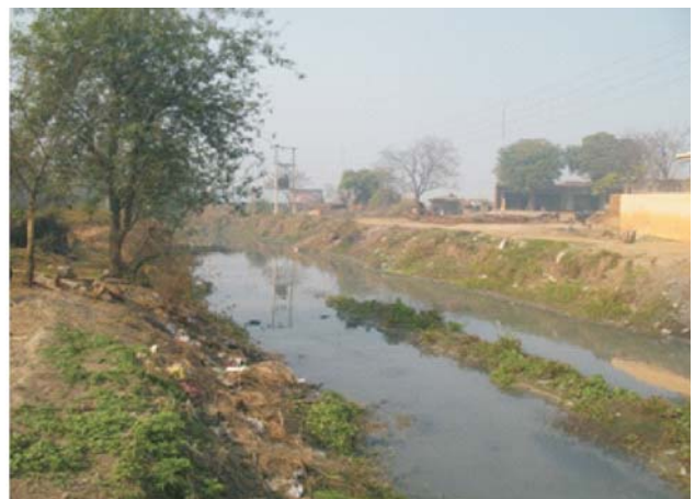
NTPC canal after removal of vegetation cover.
